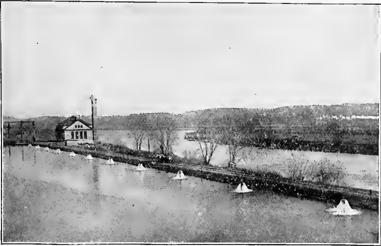
SEDIMENTATION-BASIN, PUMPING-STATION, AND OUTLETS.
